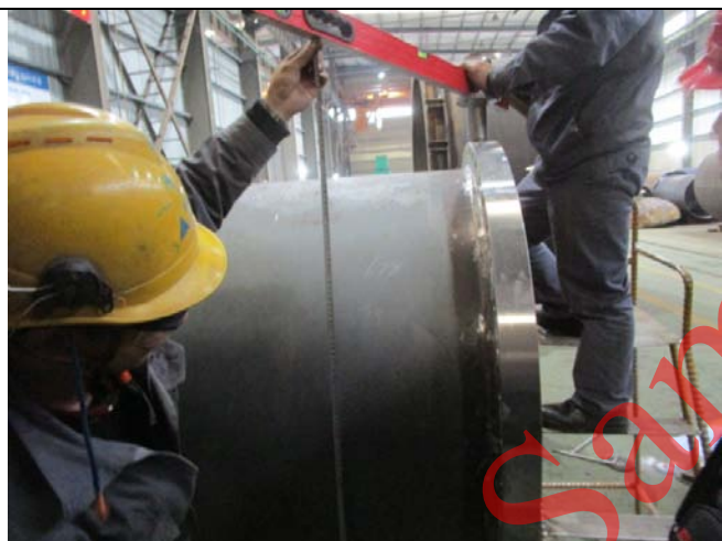
Photo 11. Fitting up check of V1&V2: tack welding parameter
